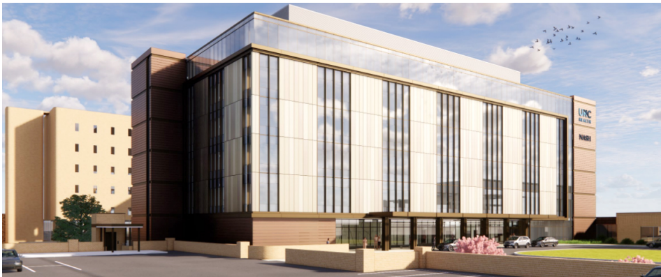
A new "patient bed tower" planned to host 150 patients, with 30 patient rooms per floor, is in the design development phase for UNC Health Nash in Rocky Mount, and new medical offices are planned for construction in Nashville and Middlesex.
